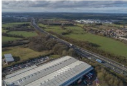
M54-M6 Link Road 81,890 tCO 2 e 1.6 miles new road 2 new junctions & some realignment
